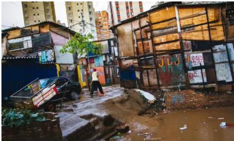
The flooding as a result of the makeshift plumbing/sewage system
